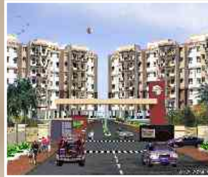
Mahalaxmipuram Phase-I Baran Road, Kota
