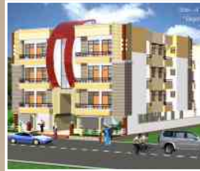
Surya Residency Near Railway Station, Kota
